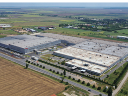
ROMANIA Romania Plant
