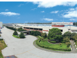
CHINA China Plant (MCC)
